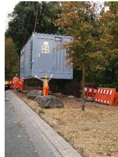
Installing the substations
