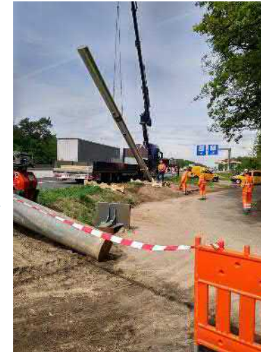
Erecting poles
