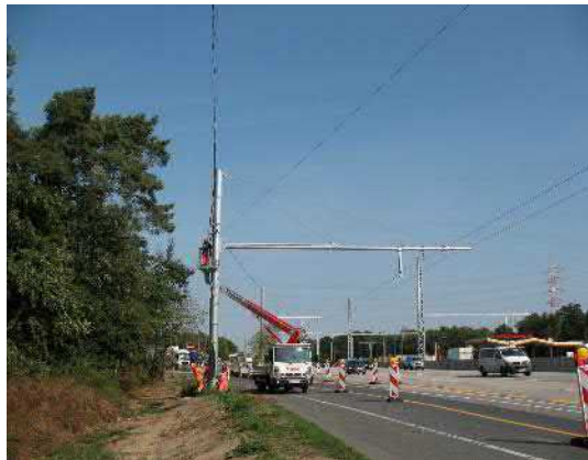
Attaching cantilevers
