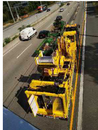
Pulling the contact line
